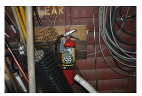
Common Types: Different extinguishers are designed to fight different types of fires. Most extinguishers are combination extinguishers, of the "ABC" type, which can be used to fight many common fires.
